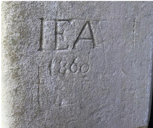
Fig 5. North chancel doorway. Dated initials
